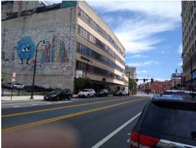
Photo 1: The Denholm building at 484 Main Street (Parcel 1).
