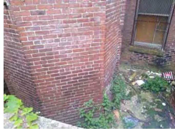
Photo 6: Base of brick smokestack on Parcel 2.
