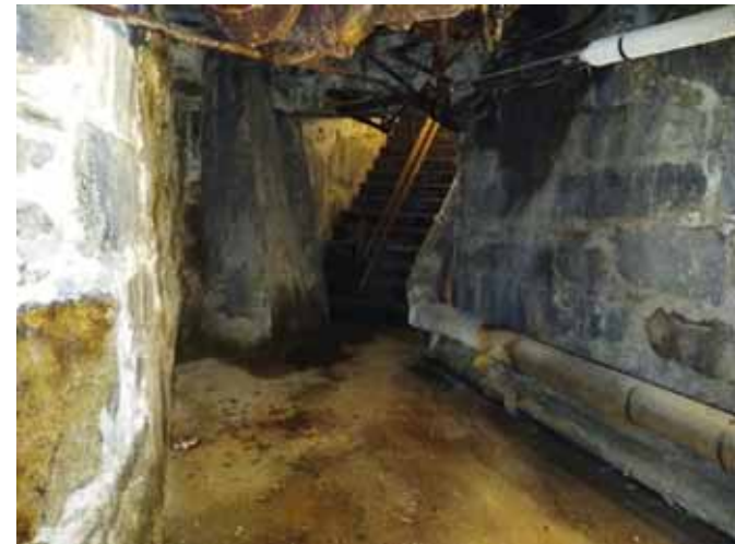
Photo 16: Passage under Chase Court connecting Parcels 1 and 2.
